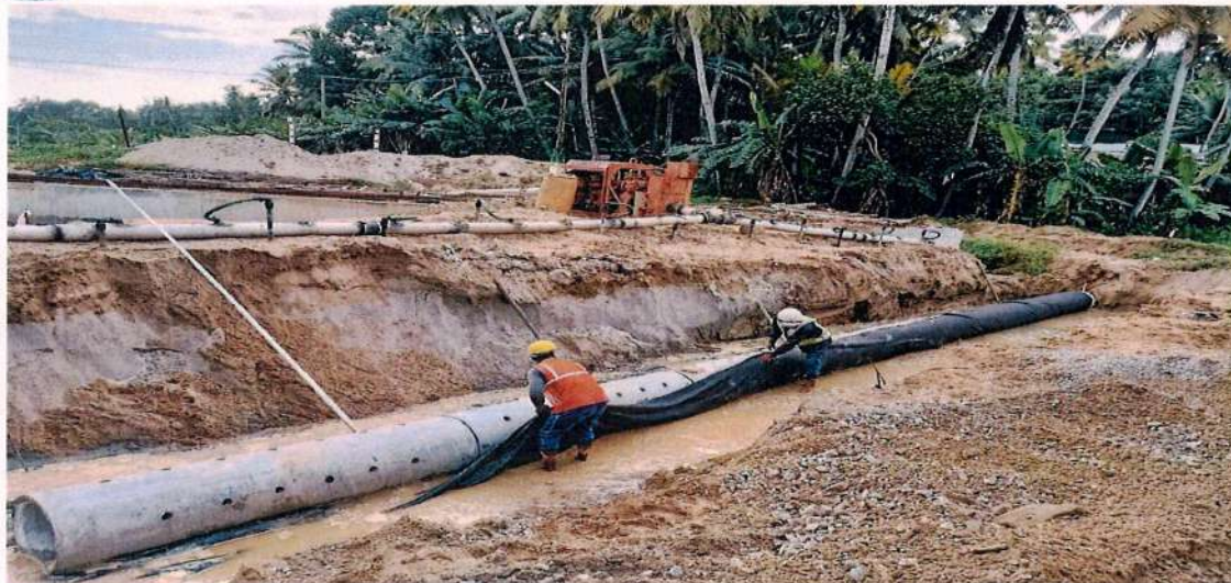
Construction of cross vents at 540 m
