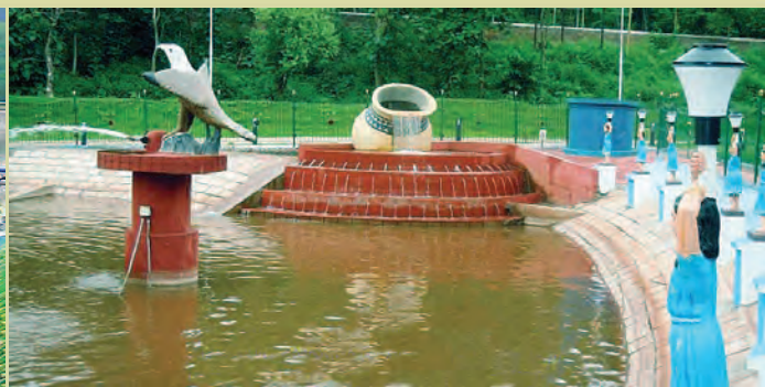
Raiwater Harvesting Pond at TATA Steel Ltd., Odisha - Capacity 30,00,000 l/day
