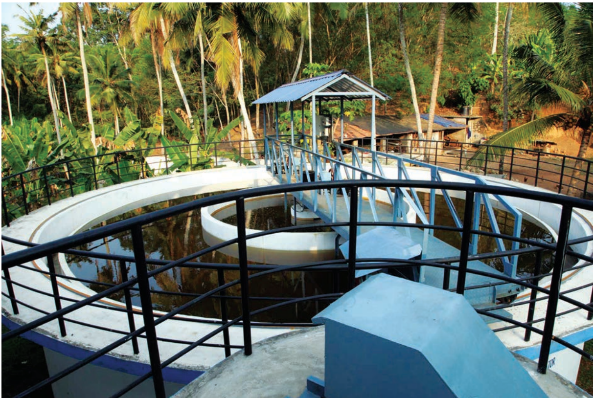
Drinking water plant
