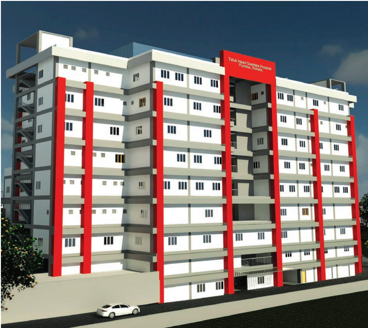
Taluk Head Quarters Hospital, Punalur(KIIFB Project)
