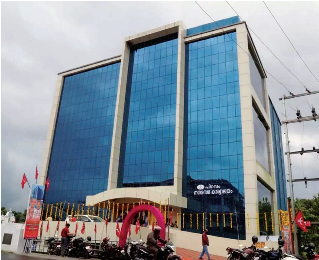
Supplyco suburban mall, Piravom
