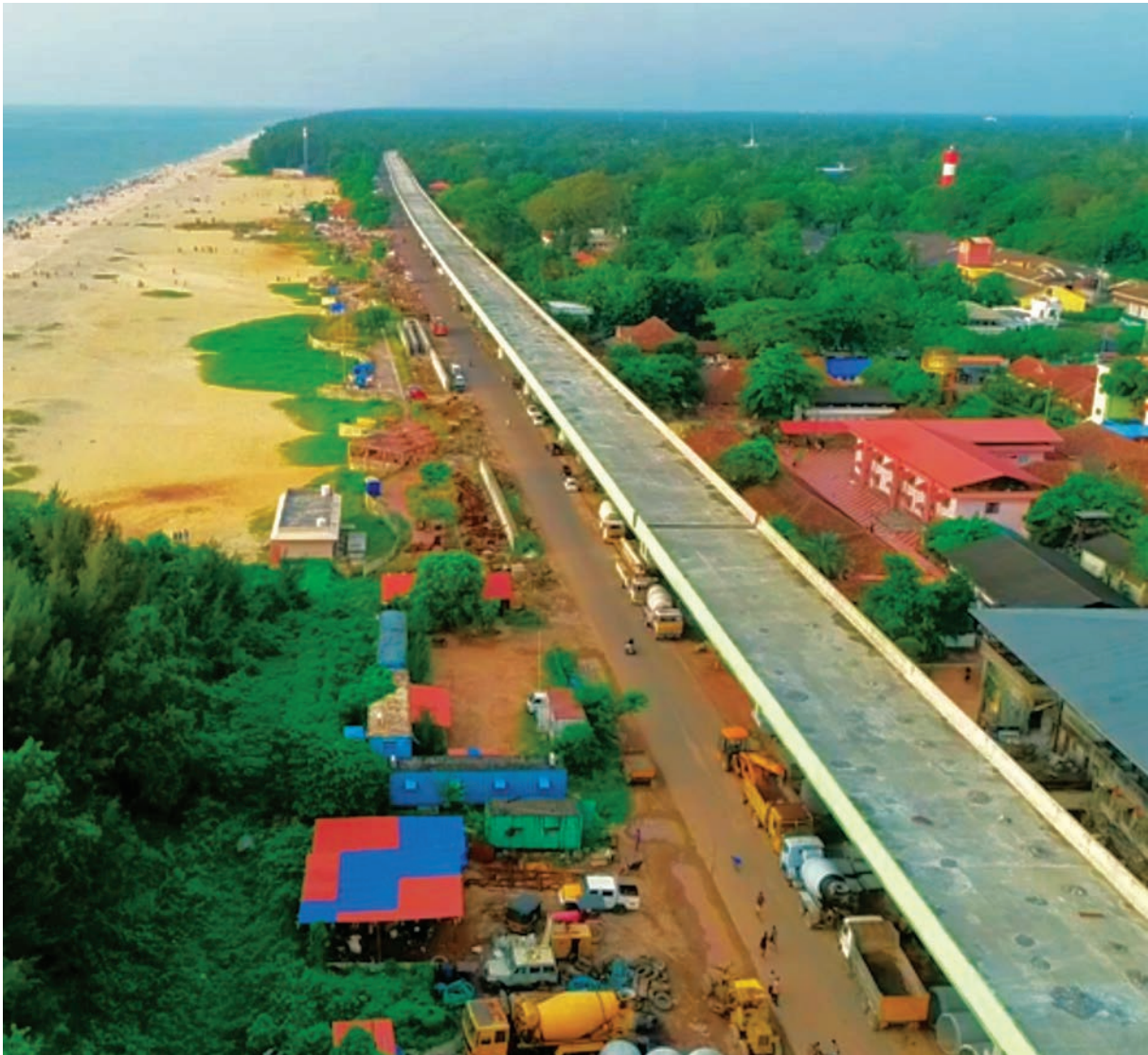
Alappuzha Bypass Aerial View
