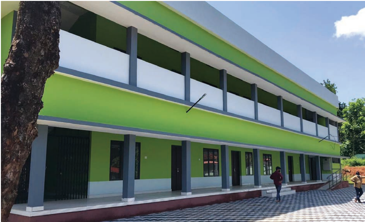
New Building for Govt. ITI Vettikavala, Kollam
