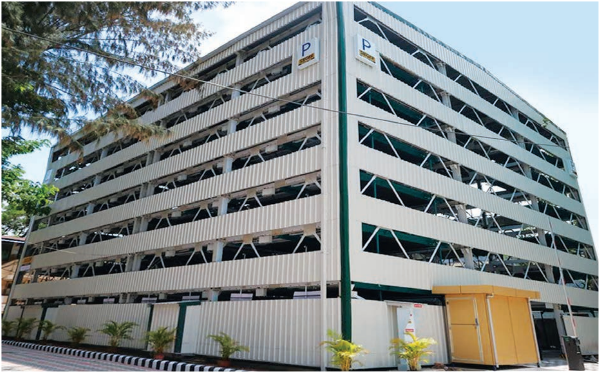
Multi level car parking , Thiruvananthapuram
