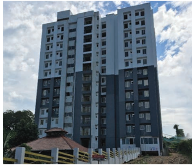
Apartment complex being constructed at Ponjassery under Janani project:
