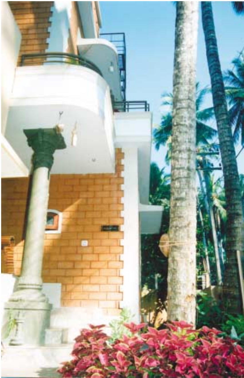
Building constructed with compressed hard brick (popularly known as interlock brick)
