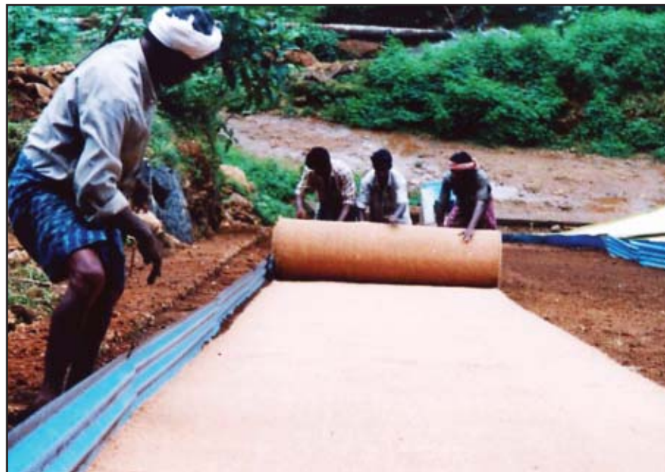
Laying of coir geotextiles
