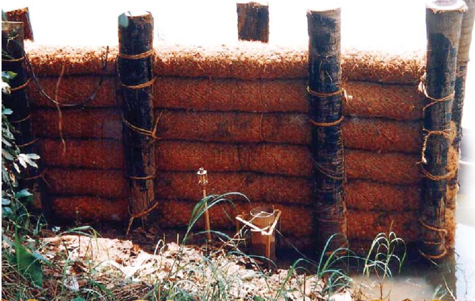
Spurs constructed with coir geotextiles (Cocologs)
